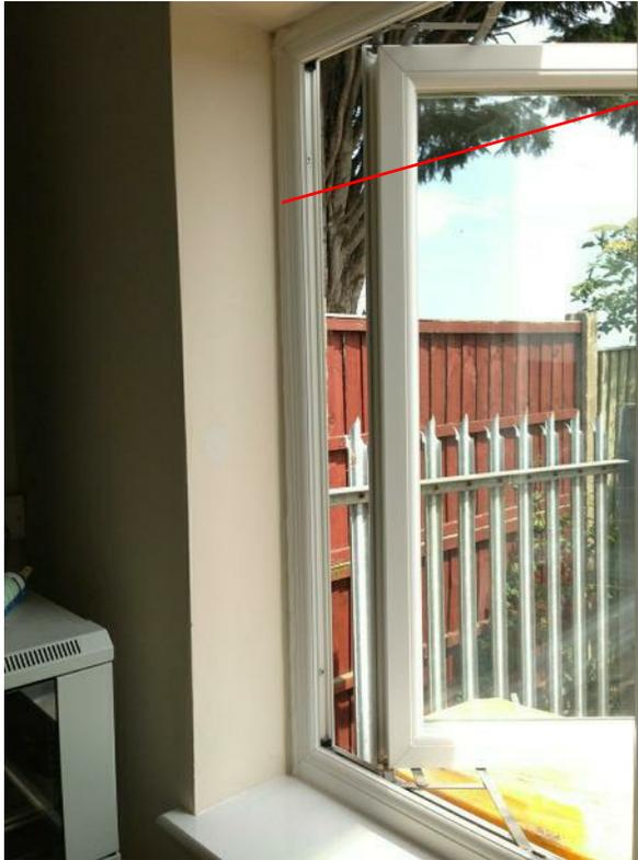
Run a 10mm bead of silicone around the top and sides of the window frame
